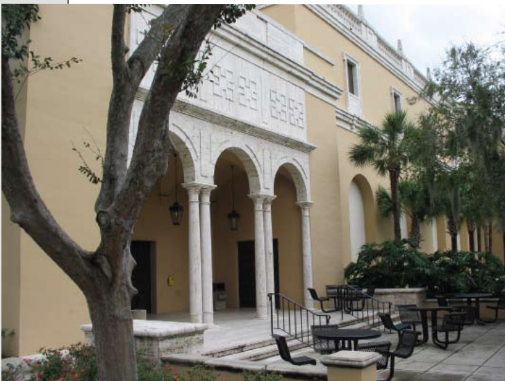
The five-level Bush Science Center at Rollins College houses a state-of-the-art multimedia classroom auditorium, a data center, and teaching laboratories. The 30-year-old building presents several HVAC design challenges.
