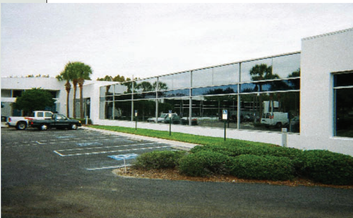
PHOTO A. This Tampa, Fla., building had windows that were unprotected from the area's frequent downpours. The windows were caulked and sealed to fix the problem (Figure 1).
