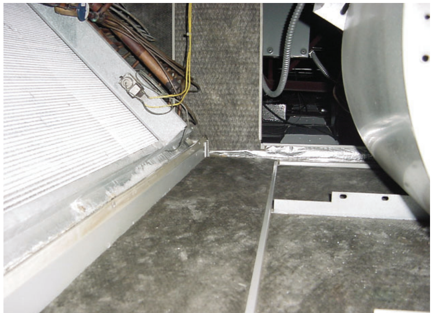
PHOTO C. Air handler disinfected and cleaned with a HEPA vacuum.
