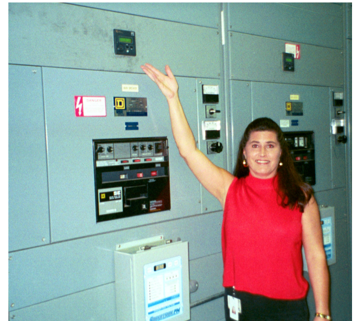
Two power monitors as installed in the main electric room at the Mid-Florida Processing and Distribution Center. The units continuously measure kW, kWh, KVAR, pf, Volts, Amps, and harmonic content.
