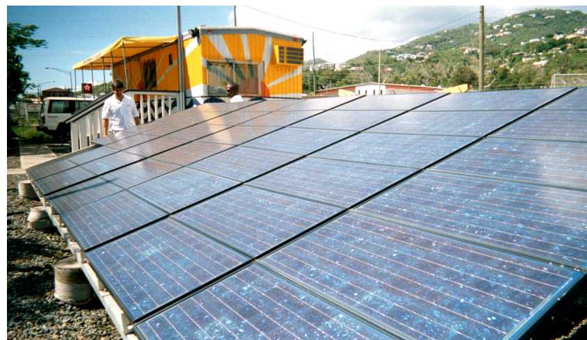
The Virgin Islands Energy Office operates a 2.5 kW demonstration solar-PV site along the main road from the St. Thomas airport to the cruise ship docks in Charlotte Amalie.
