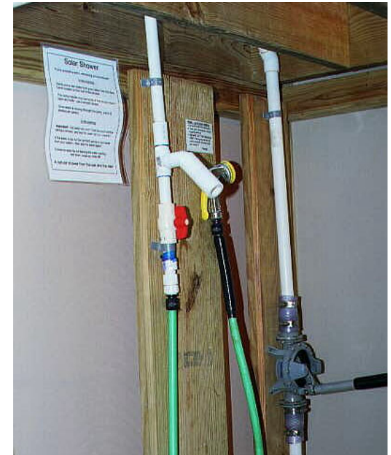
This solar shower needs a 2.5 gpm head.
