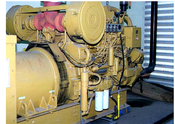
Almost every building of any size is equipped with a Diesel or LNG back-up electric generation set.
