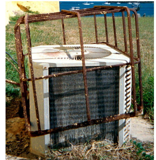
This deteriorated low-efficiency condensing unit at Ft. Christiansted should be replaced with a unit rated at SEER 12 or higher unit (2-tons).
