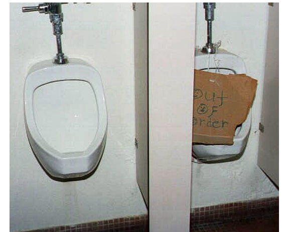
Replacement of wall-hung 3.0 gpf or 1.0 gpf units with waterless models is a significant water saving opportunity at all Federal sites visited.
