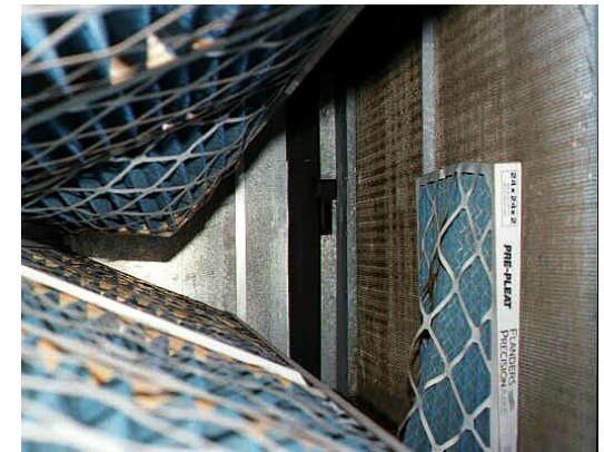
A missing filter was blown against the evaporator coil, allowing unfiltered air to foul the coil.
