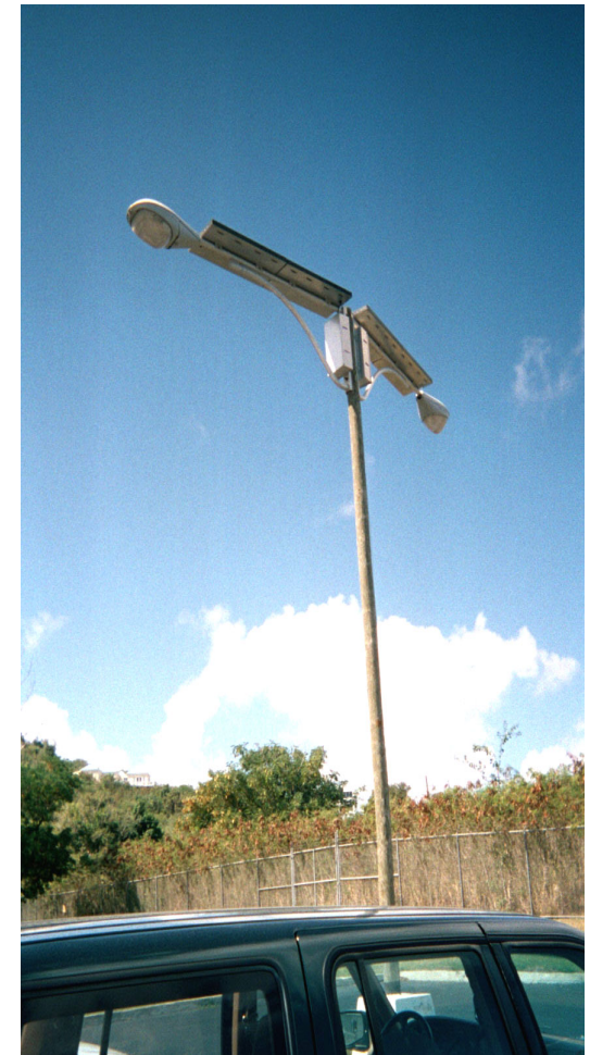
Solar PV parking lot lighting near the St. Croix federal building.
