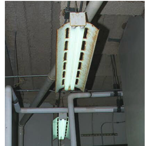
Inefficient T12 light fixtures at Ft. Christiansted need upgrading to modern T8/electronic ballast fixtures.
