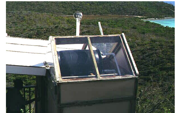
A solar hot water heating tank.
